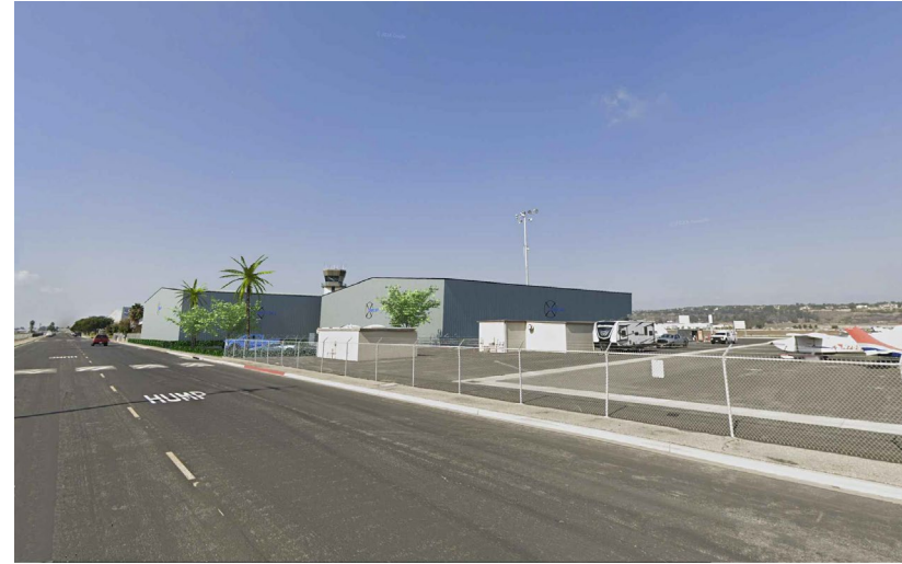
View of New Hangars from Aviation Drive
