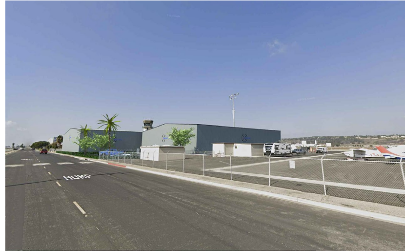
View of New Hangars from Aviation Drive
