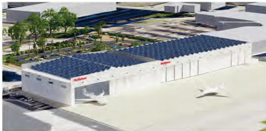
Sky Harbour – SJC Phase 2 in pre-development with rooftop solar panels
