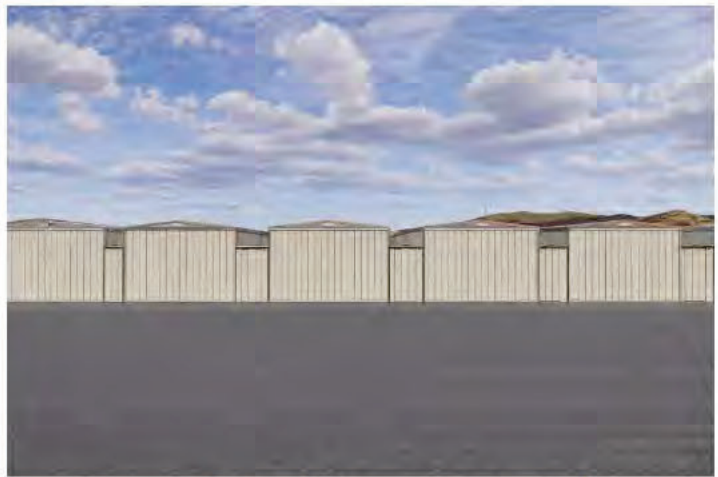
Restored T-hangars façade view 1
