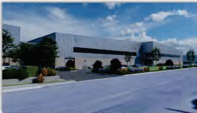
Figure 8. Aviation Drive Public Landscaping.
