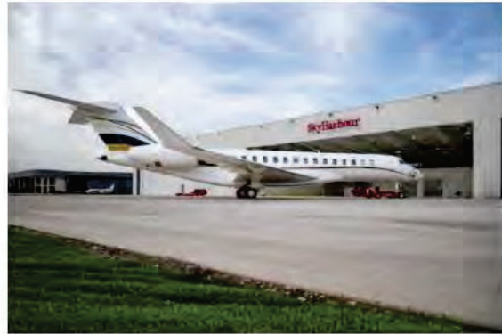
Sky Harbour - ADS Phase 1, Operational
