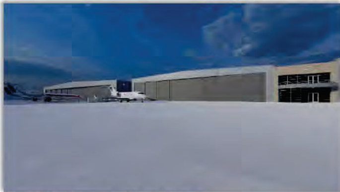
Figure 7. Air 7 Campus at CMA with Hangar 3.
